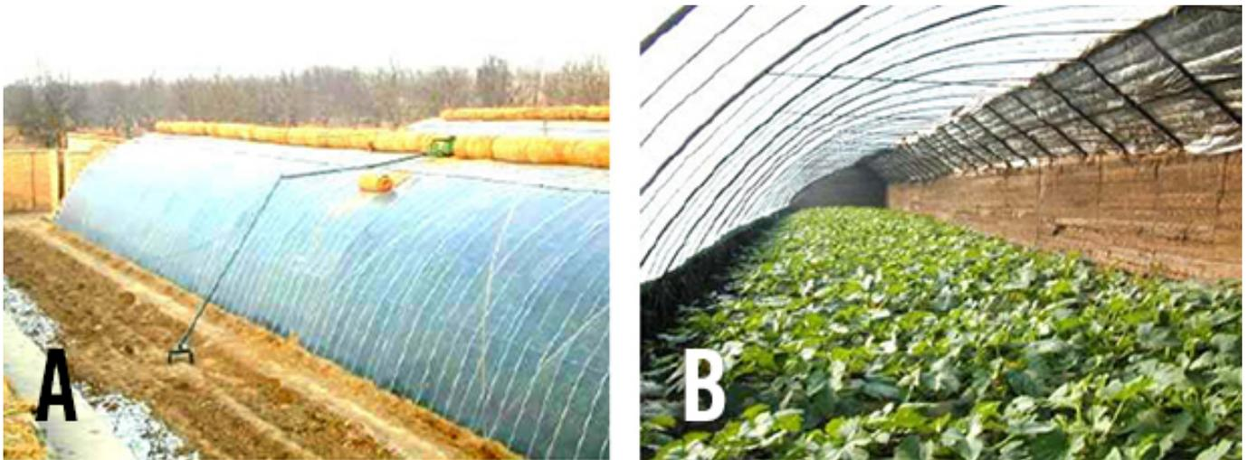
Figure 2. A Typical Solar Greenhouse in China. View A features natural grass insulation and View B shows an earthen wall for retaining heat. Photos: John Snyder, professor emeritus, University of Kentucky.
