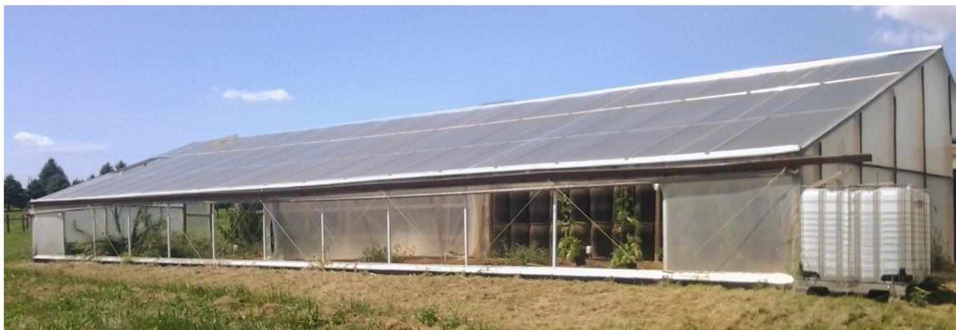
Figure 7. The South Face of the Completed Structure. A gutter was added for rainwater collection. Plastic sheeting was added to the bows on either end of the structure, similar to a high tunnel, to prevent air loss during cold periods.
