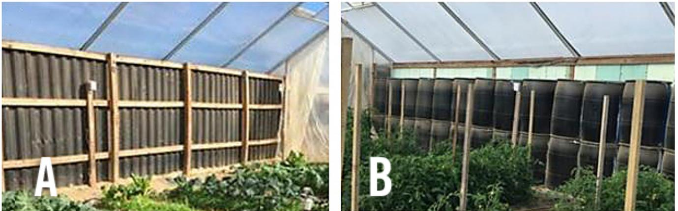
Figure 5. Two Options for Thermal Mass. A. The completed interior with the sand-filled thermal mass on the west side of the structure. B. The east side of the PSG contained stacked barrels filled with water. It may not be visible in the picture, but the barrels are secured in place with high-strength cables that are anchored to each post to prevent shifting or falling. Each barrel weighs more than 450 lb when full.
