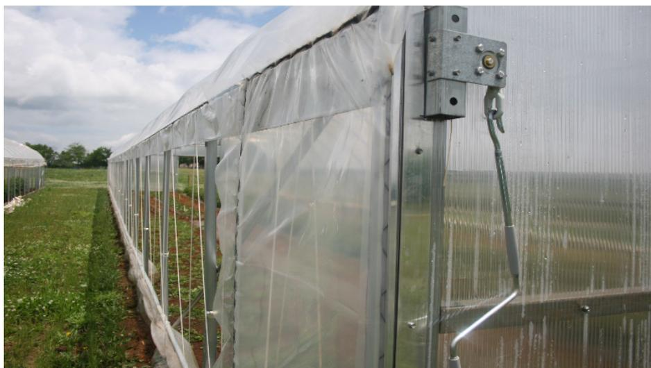
Figure 8. A Typical Sidewall From a High Tunnel Structure (with ground posts for anchoring). This type of sidewall could be
